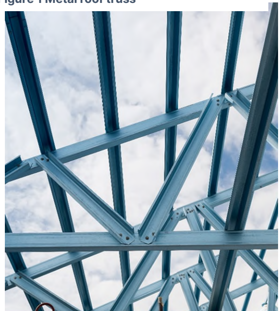
Figure 1 Metal roof truss
