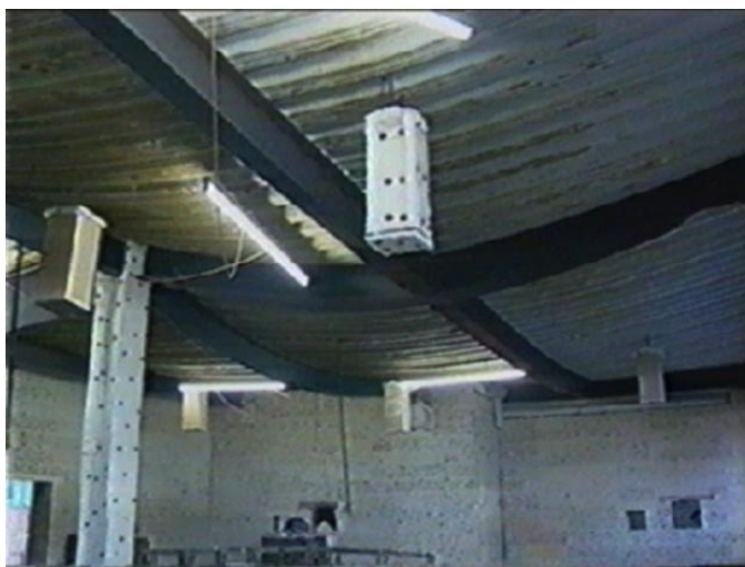
FIGURE 12.6 THE FLOOR SYSTEM AFTER CARDINGTON FIRE TEST
