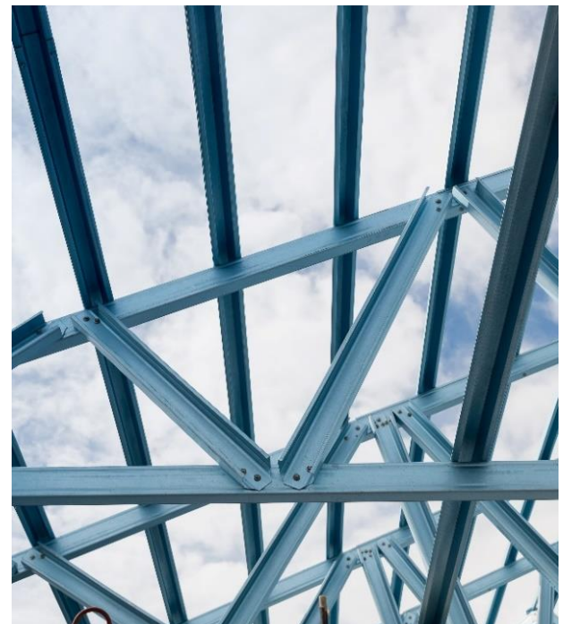
Figure 1 Metal roof truss
